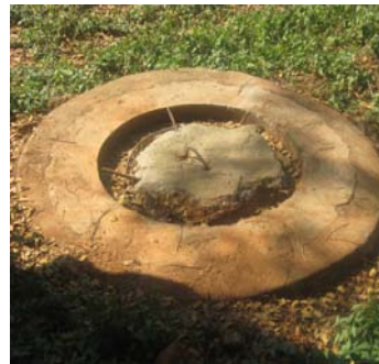
Existing Condition of Manhole
