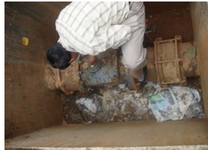
Inspection of Chamber
