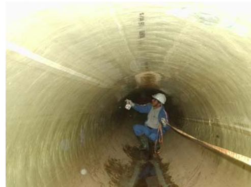
CIPP lined 1200mm Dia Sewer
