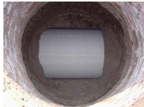
1200mm Dia CIPP liner through a manhole
