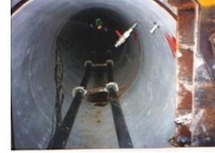
Jacking is in progress
