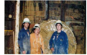
On completion of 35m deep drive
