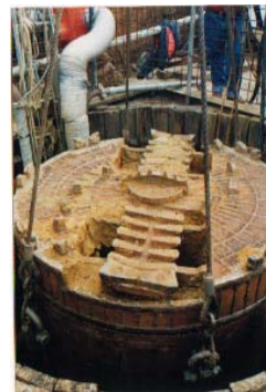
Shield is being recovered through a 3.5m dia receiving shaft
