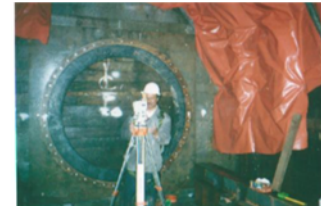
Setting up at 35 m deep shaft
