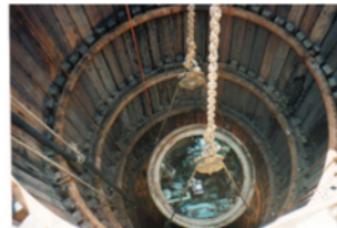
Lowering of 1500mm dia shield
