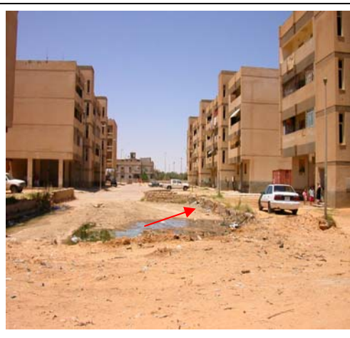
Existing Drainage System
