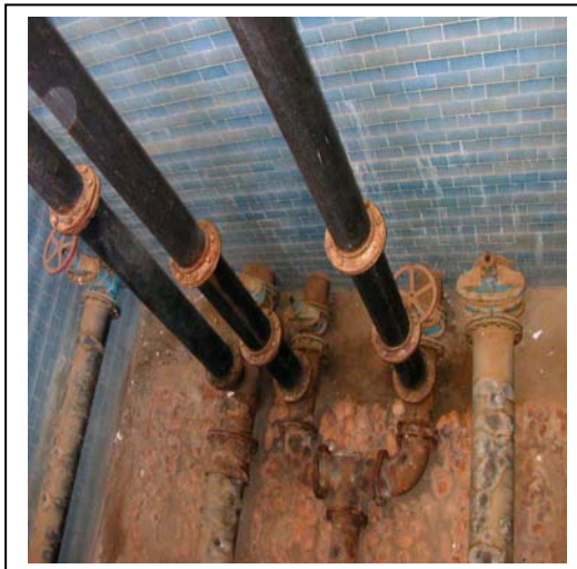
Existing outlet pipes
