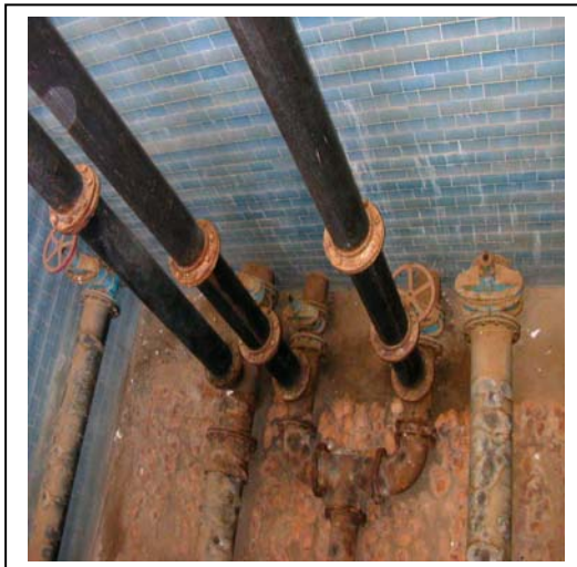
Existing outlet pipes
