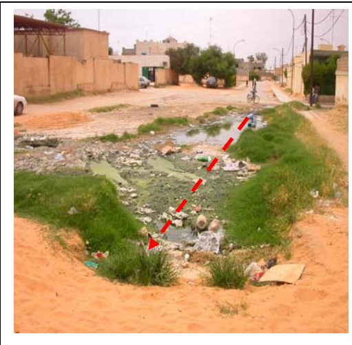
Existing Sewerage System
