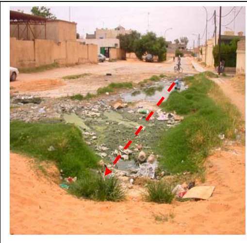
Existing Sewerage System
