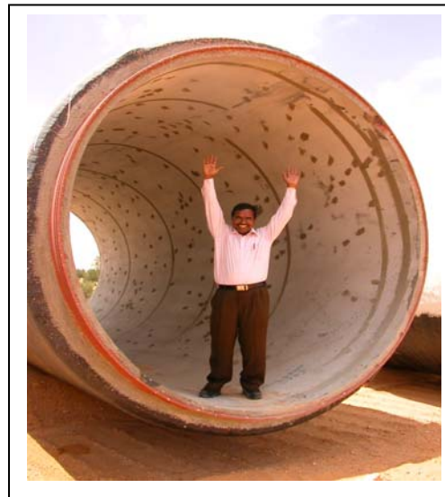
3000mm Dia Pipe in GMMR
