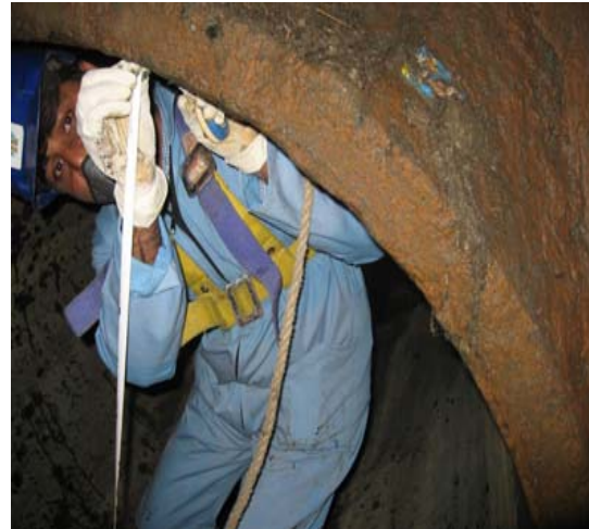
Internal Measurement of Pipe Diameter
